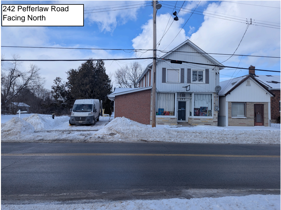
242 Pefferlaw Road Facing North
