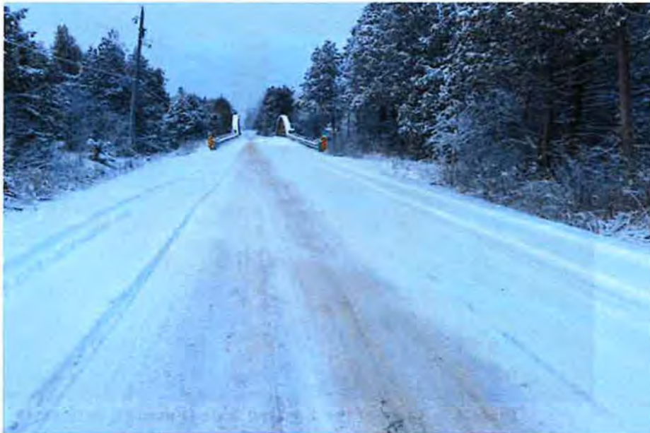
Plate 2 View of East Approach (Facing West)
