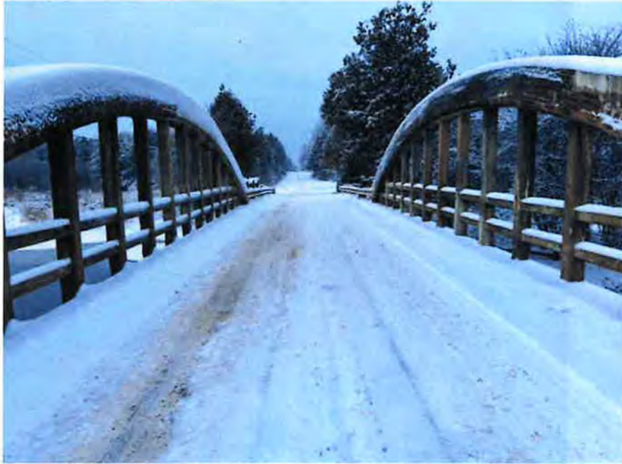
Plate 5 View of Deck (Facing West)
