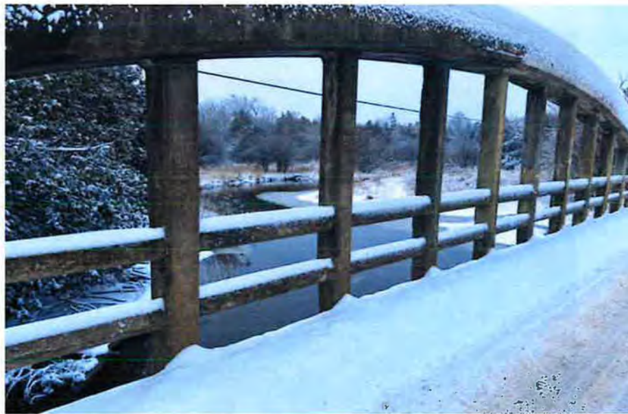
Plate 4 View of the Eastern Side (Facing Southwest)
