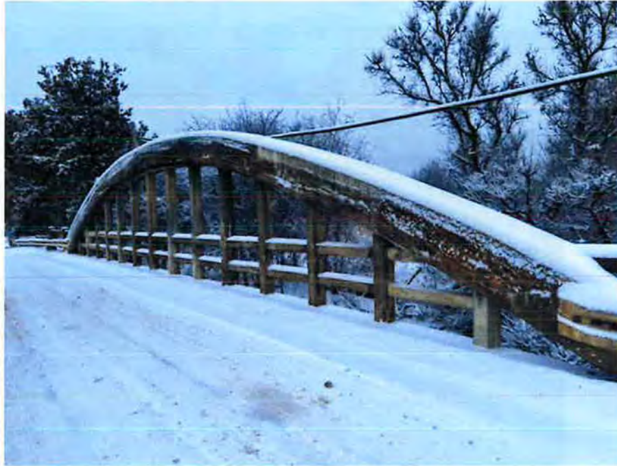
Plate 3 View of Deck (Facing Northwest)
