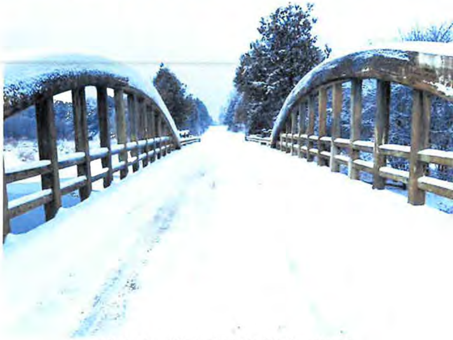
Plate 5 View of Deck (Facing West)
