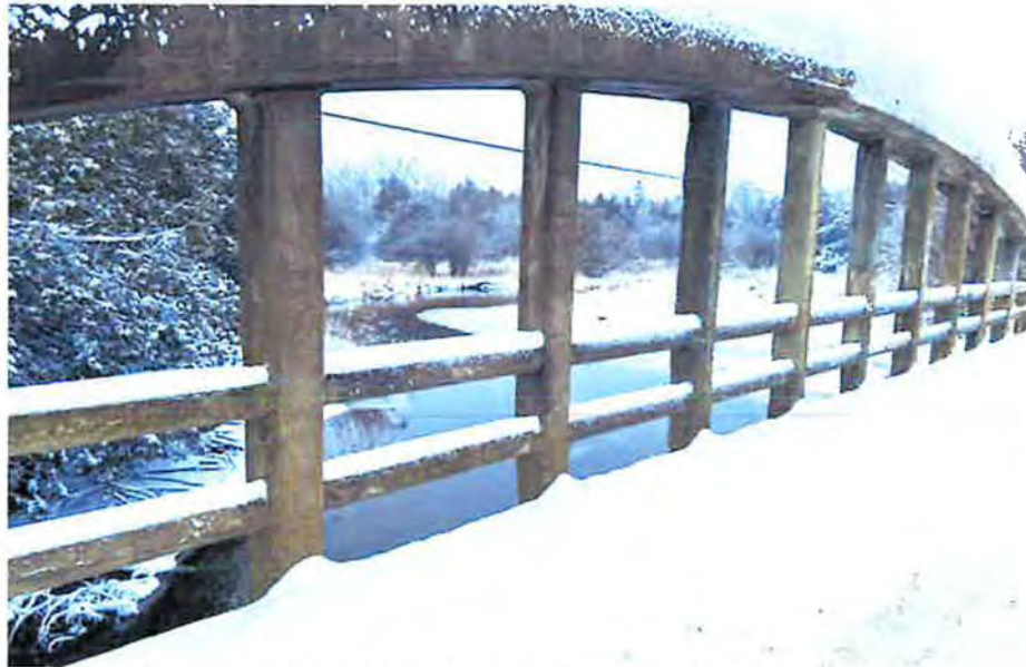
Plate 4 View of the Eastern Side (Facing Southwest)
