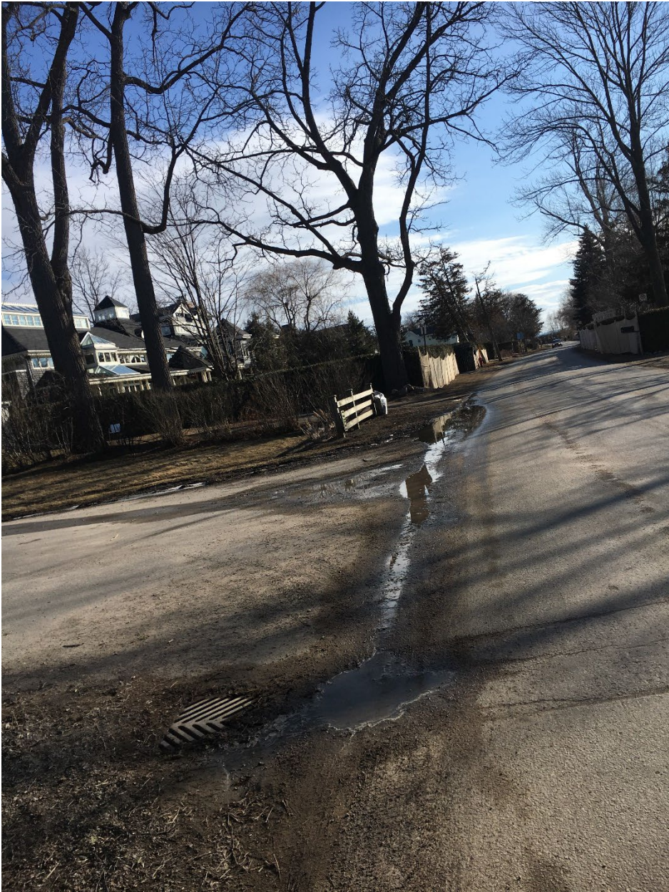
Photo 3: shows the culvert where the water from the rear of 255 Lake drive north east beyond Metro road used to be diverted. The water now flows predominantly in front of 253A and some to 253 Lake drive North
