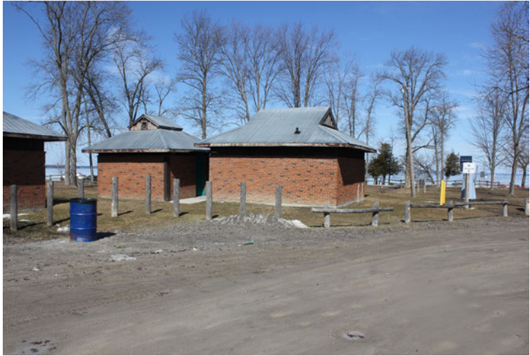
Existing washrooms/change rooms in Willow Beach Park
