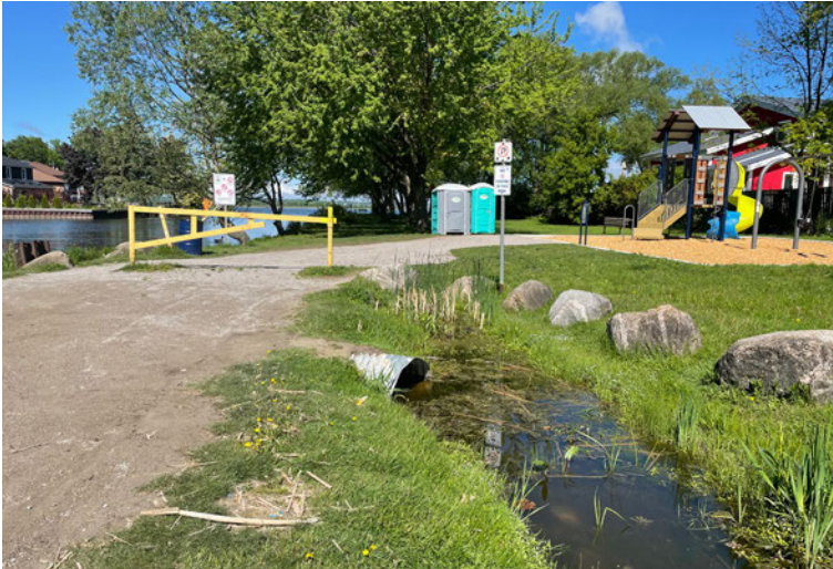
Playground and drainage culvert
