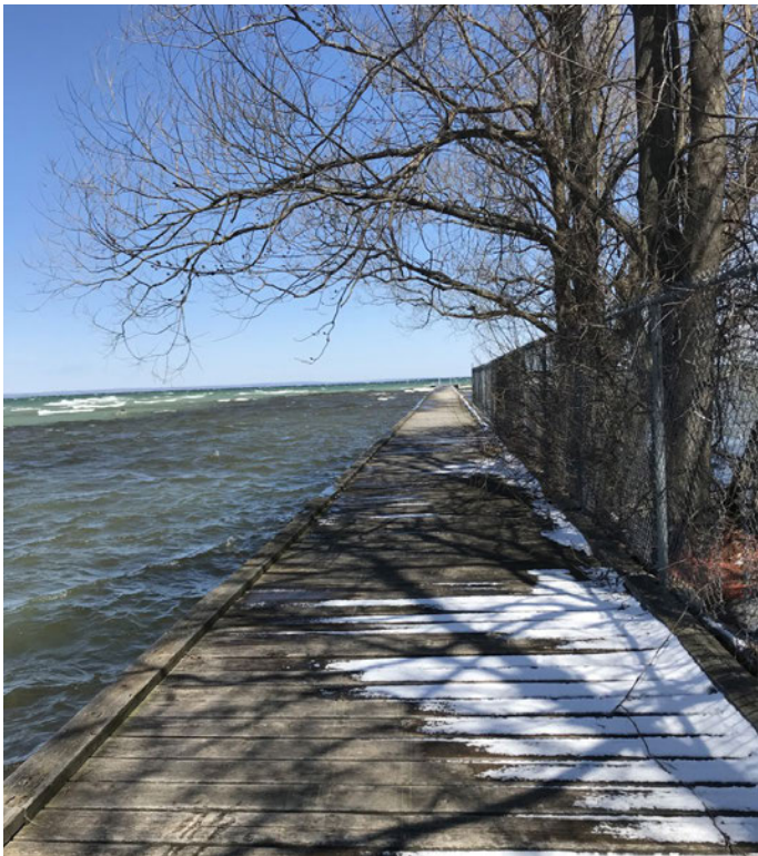
Existing shoreline conditions at Mossington Wharf
