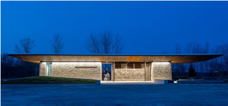
Stanley Park, Toronto Washroom
