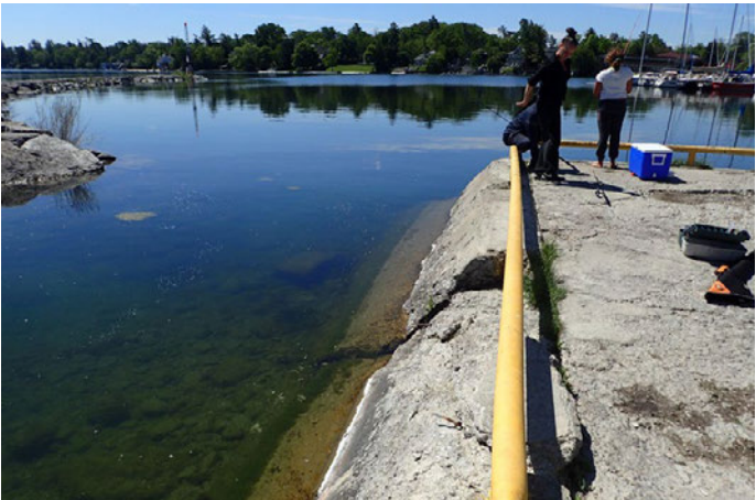
Existing shoreline conditions along Malone Wharf
