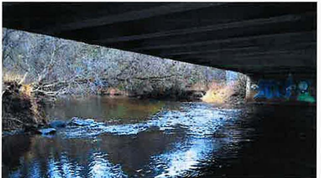
Photo 6. Facing northeast from underneath bridge.
