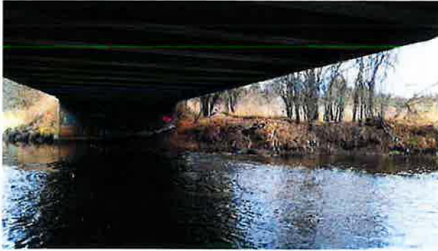
Photo 7. Facing west underneath bridge.
