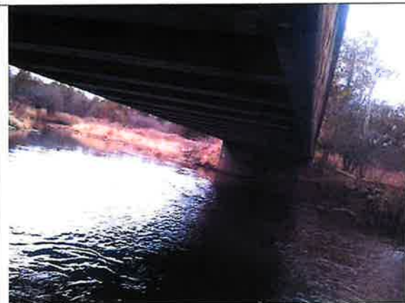
IMAGE 5 UNDERSIDE OF OLD SHILOH BRIDGE EAST
