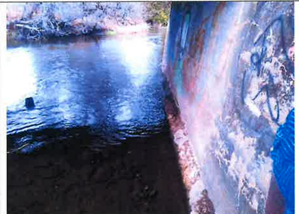
IMAGE 6 CONCRETE PILASTER OF OLD SHILOH BRIDGE EAST
