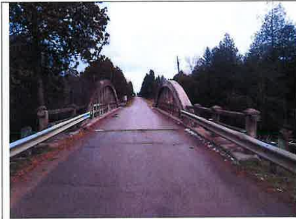
IMAGE 1 VIEW OF OLD SHILOH BRIDGE EAST
