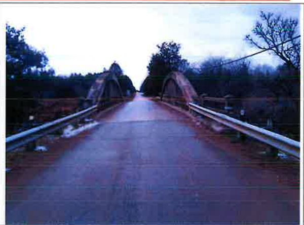
IMAGE 8 OVERVIEW OF OLD SHILOH BRIDGE EAST
