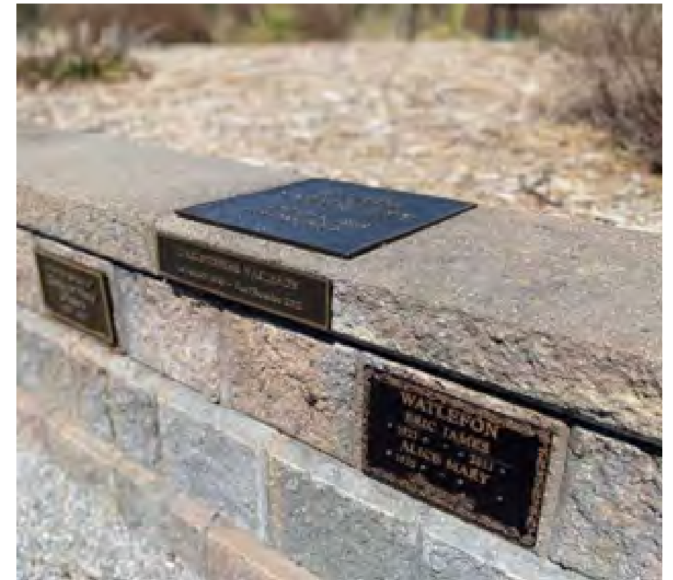
Figure 21: Bronze Memorial Plaques, mounted on a Modular Concrete Block Wall at Keswick Cemetery, Source: LEES+Associates, 2023.
