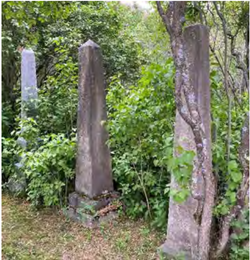
Image: Vegetation encroaching on monuments at Mann Cemetery. Source: LEES+Associates, 2023.
