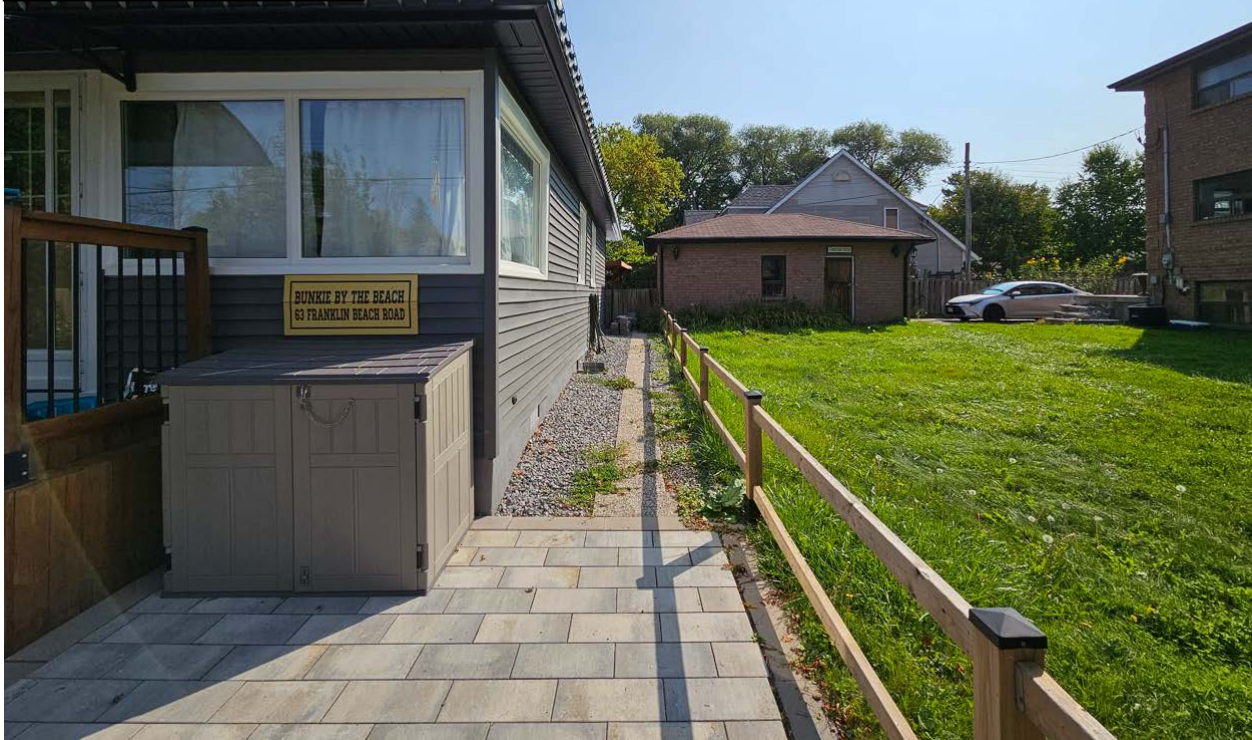
63 Franklin Beach Road Facing East
