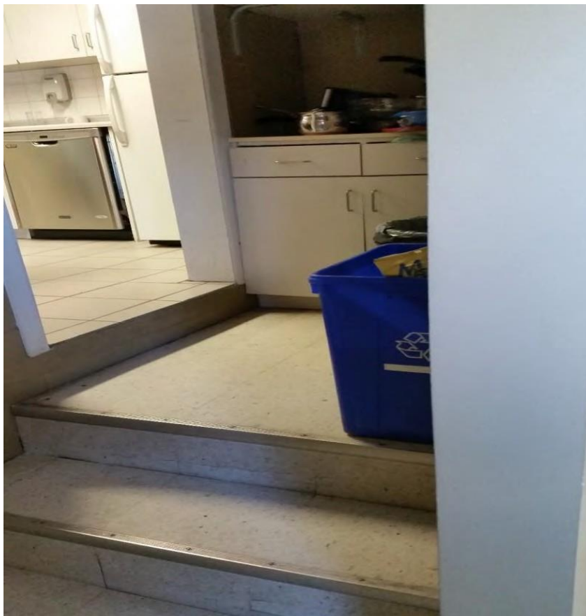
(photo: only exit from the crew dormitory through the kitchen)
